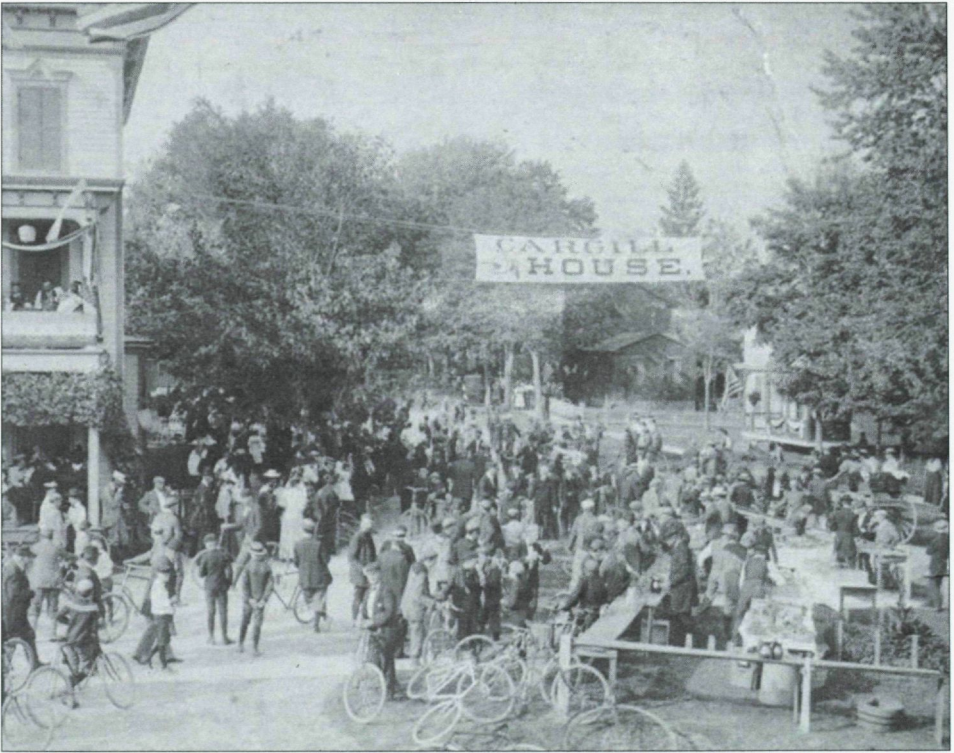
Pictured here is the end of the Scottsville line of the Monroe County sidepath system. It is likely that this picture was taken on opening day of the Scottsville line. The Sidepath Guide reported that official opening of the path “was an event in the lives of the Rochester wheelmen and wheelwomen who rode to Scottsville on that day, and to the Scottsville people it was the greatest event in years. The hospitality which was extended to the visitors was unlimited. Barrels of lemonade, with wagon-loads of edibles were distributed to the hungry wheelmen from tables in the village square.” Photograph courtesy of the Rochester Public Library, Local History Division.
